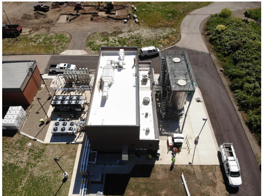
Birds-eye view of the RNG facility at the wastewater treatment plant
