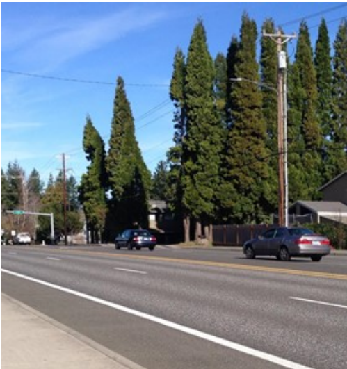
Kane Road porous overlay test project 10 years after installation.
