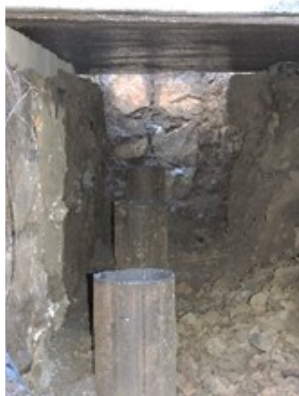
Figure 3. Tight fit behind existing abutment.
