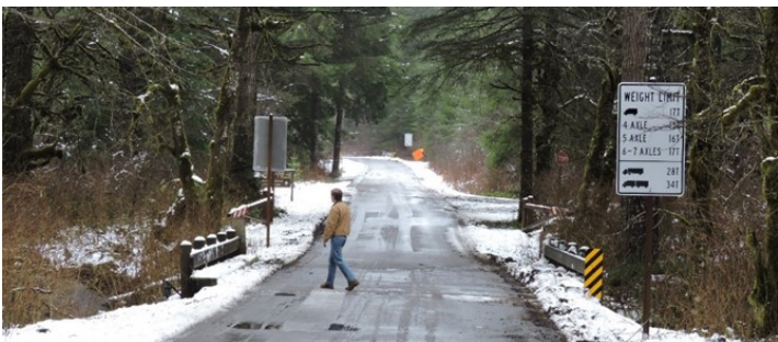
Figure 1. Corridor prior to the project.
