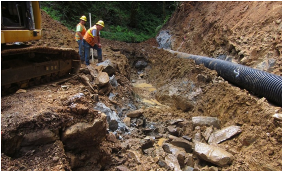
Figure 5. Material at foundation elevation.
