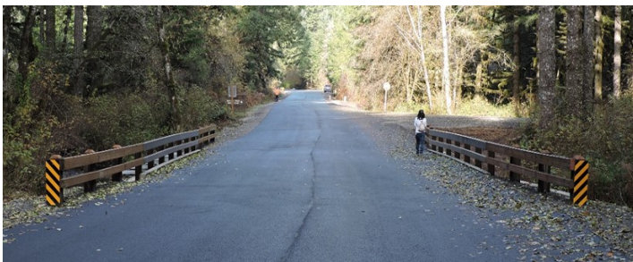
Figure 4. Corridor after project completion.
