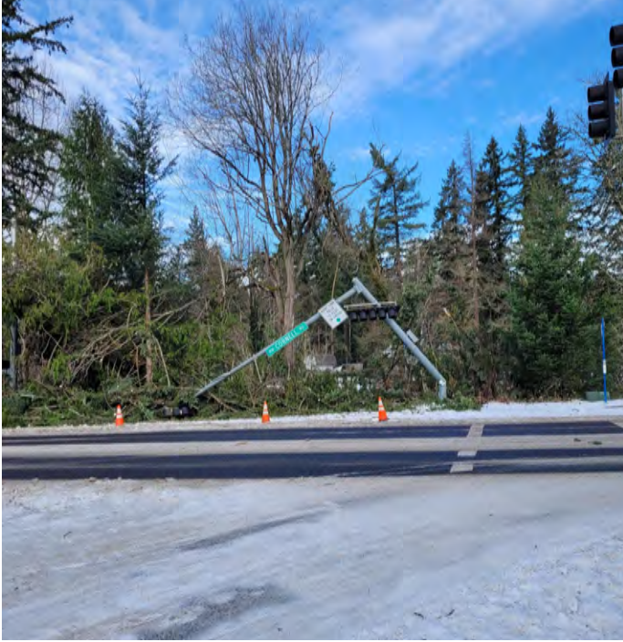
A traffic signal pole was crushed by a tree falling in Washington County so a temporary span-wire repair was put in place to get the signal back up and running until crews are able to get a replacement pole.
