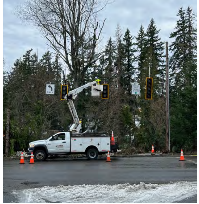
A traffic signal pole was crushed by a tree falling in Washington County so a temporary span-wire repair was put in place to get the signal back up and running until crews are able to get a replacement pole.
